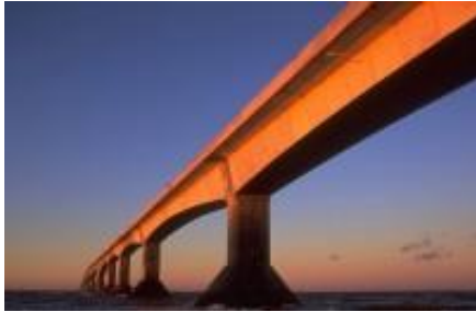
The Confederation Bridge is 12.9 km long, the longest bridge in the world crossing ice covered water. The bridge opened to traffic in the spring of 1997, ending 70 years of daily ferry service.
