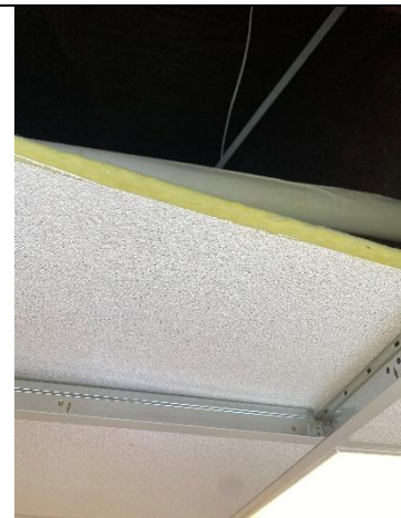
P2 – dotted ceiling tiles (fiberglass)
