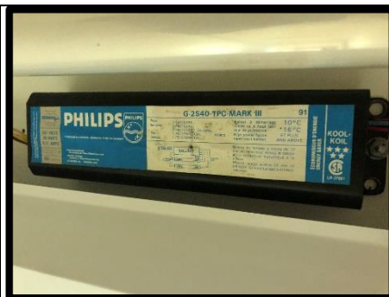
Photo 1 – Philips Mark II ballasts (Non PCB)
