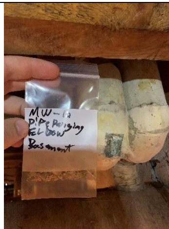
ACM Parging cement on pipe fittings
