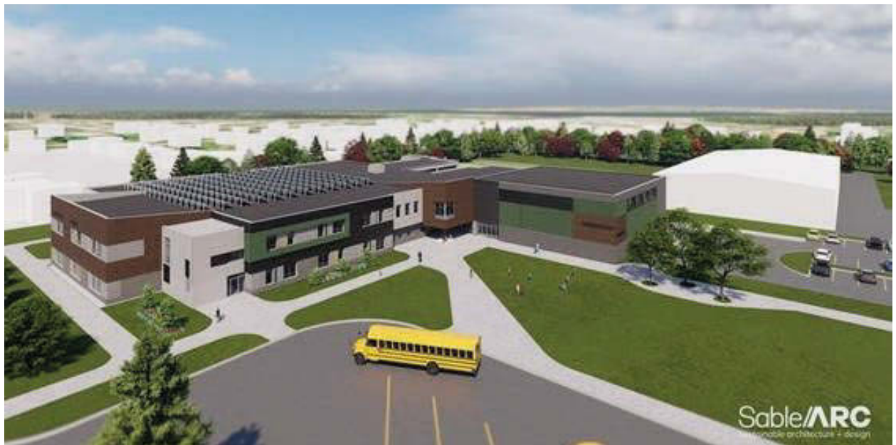
Cardigan Consolidated and Sherwood Elementary schools in Prince Edward Island are the first in the province to receive net-zero upgrades, including solar and geothermal technology.
