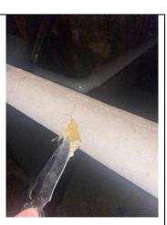
Straight run fiberglass insulation
