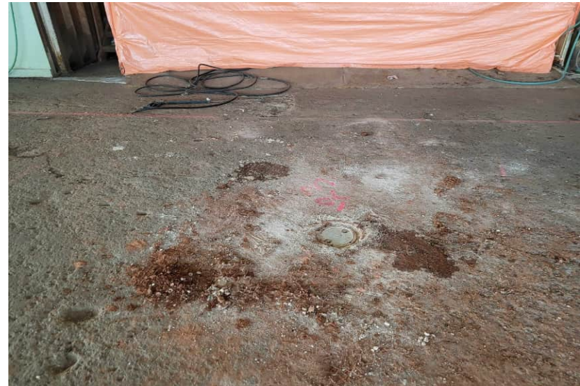
10. Looking towards MW23-23.
