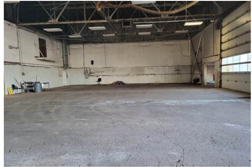
6. Looking west across the interior of the garage.
