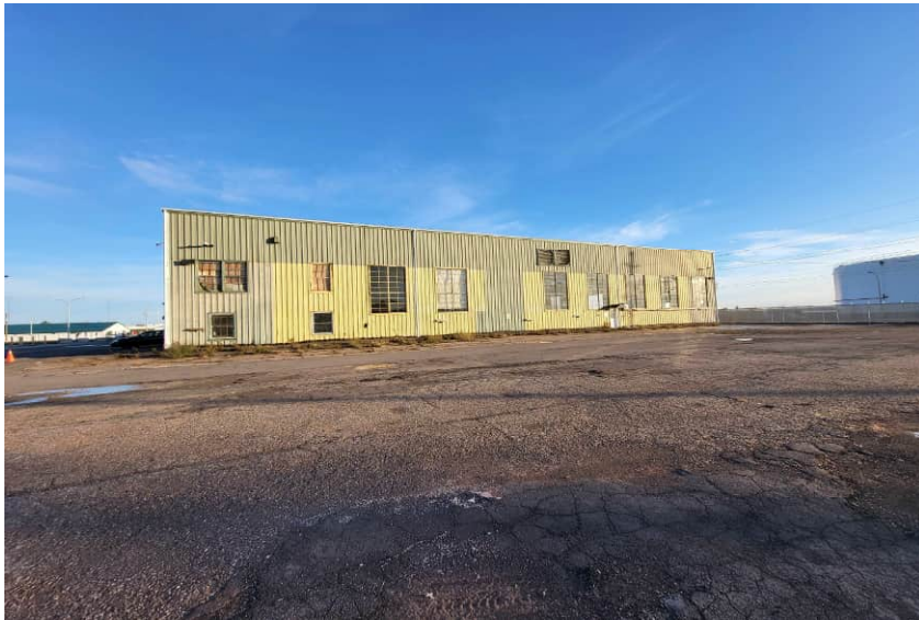
3. Looking north towards the south side of the government garage building.
