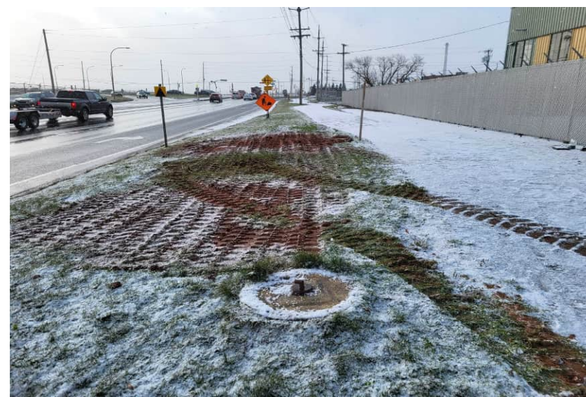
16. Looking south towards the backfilled test pit locations.
