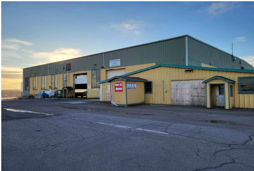
1. Looking southeast towards the north side of the government garage building.
