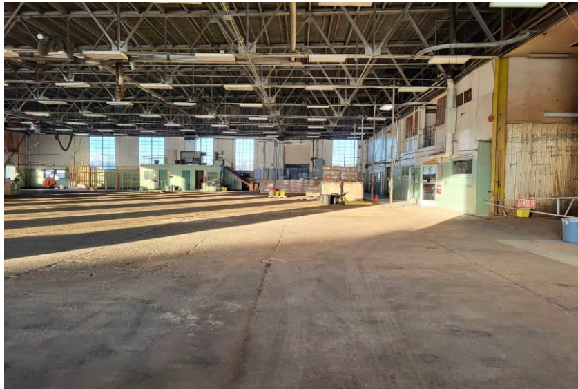
7. Looking west across the interior of the garage.
