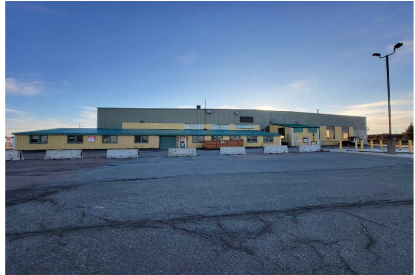
2. Looking east towards the west side of the government garage building.
