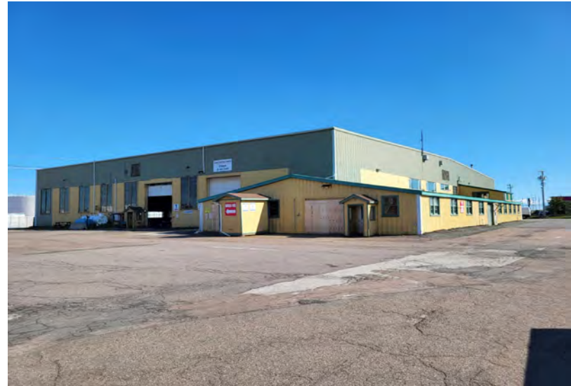
2. Looking southeast towards the government garage building.
