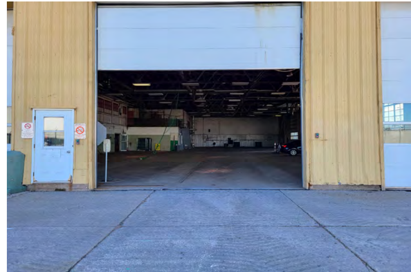
10. Looking west towards the interior of the government garage.
