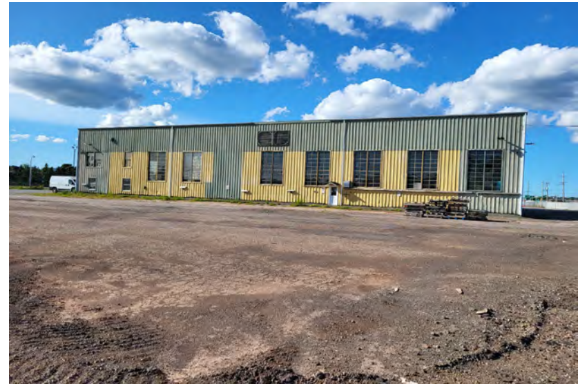
6. Looking north towards the south side of the government garage building.
