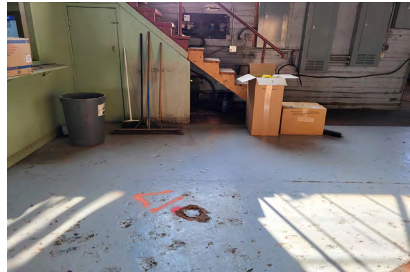
12. Looking west towards BH23-17
