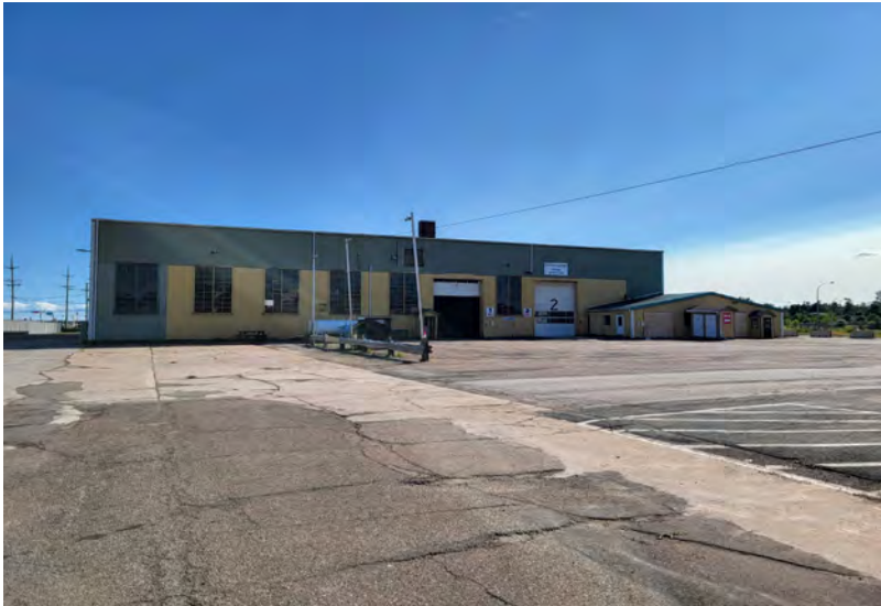
1. Looking southwest towards the government garage building.
