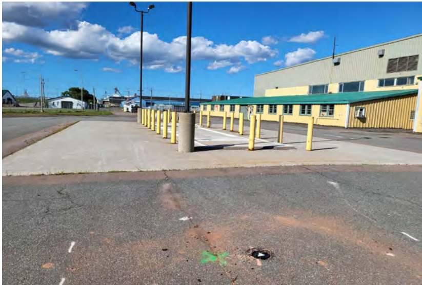
5. Looking north towards the former tank farm.
