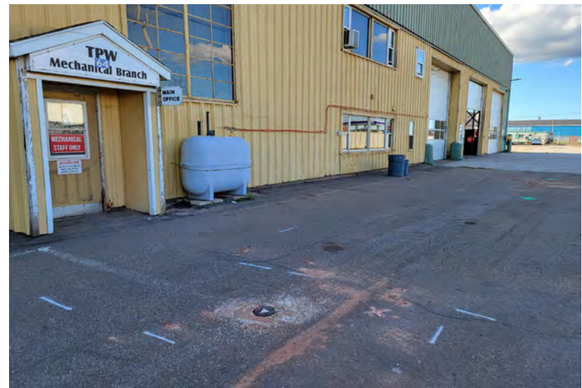
8. Looking northwest towards MW23-12, active AST, and former pump island location.
