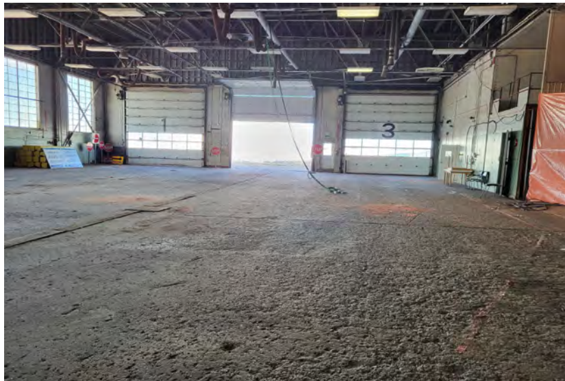
11. Looking east across the interior garage bay area.
