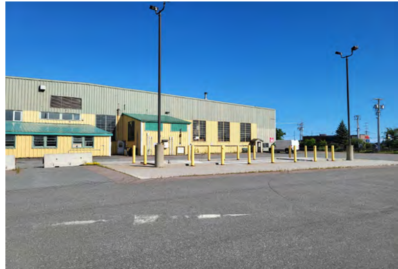
4. Looking southeast towards the government garage building and former tank farm.
