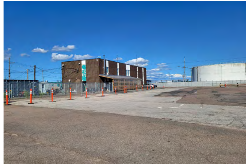
14. Looking northeast towards the administrative building.
