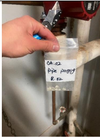
Parging cement on pipe fittings
