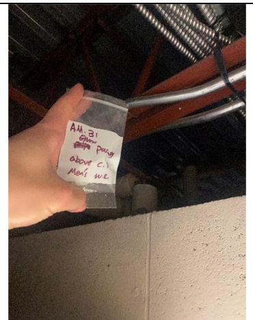
Parging cement on pipe fittings (above ceiling tile)
