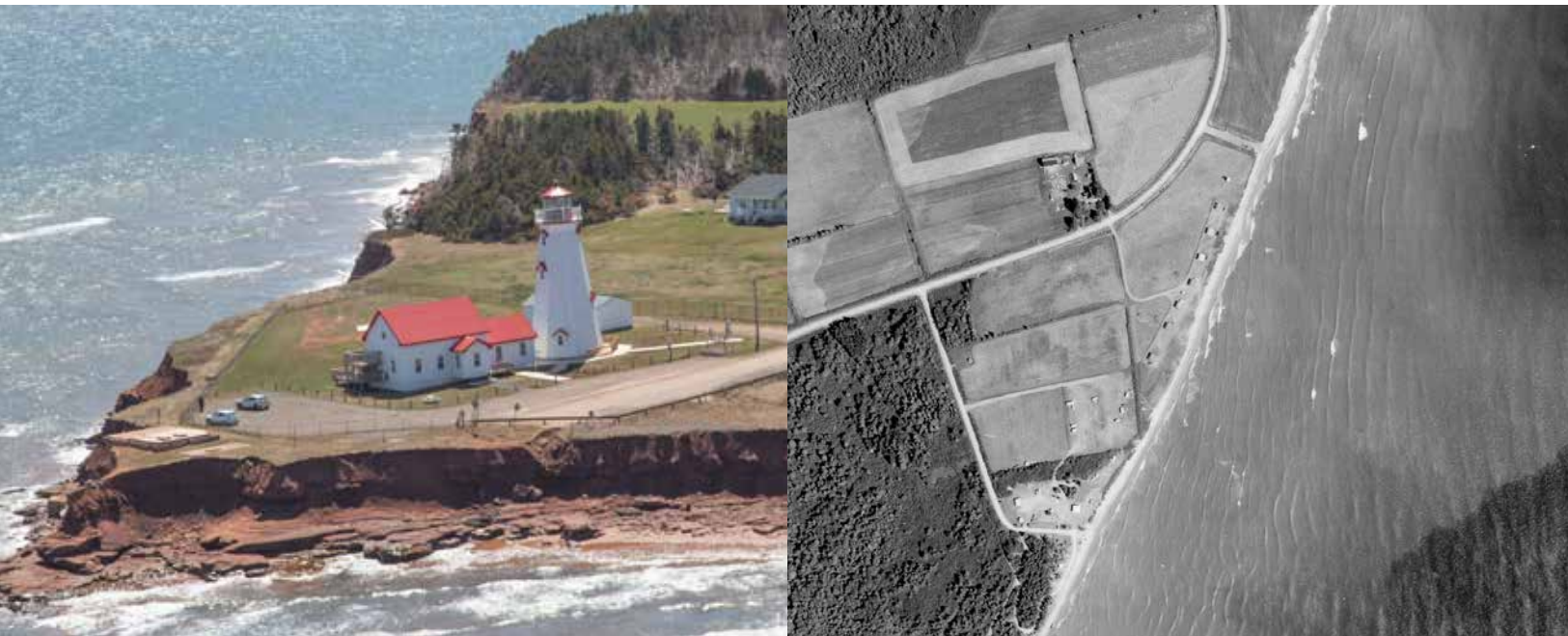
Figure 2. (left) East Point lighthouse with remnants of the previous foundation location at the edge of the bank (D. Jardine, 2023)
