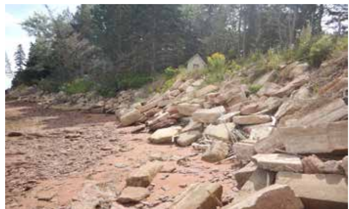
Figure 68. Typical residential shoreline armoring with old concrete/construction debris (H. Parnham, 2018)
