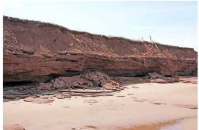
Figure 29. Cliff undercutting at Lower Darnley (D. Jardine, 2011)
