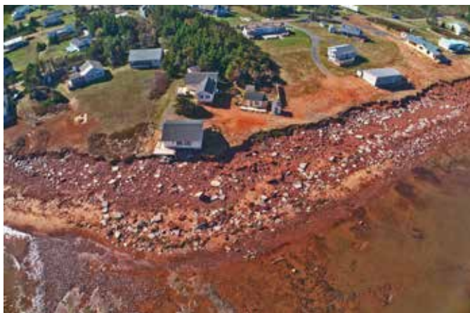
Figure 27. Coastal erosion and property damage at Savage Harbour, Pigots Point (UPEI, 2022)
