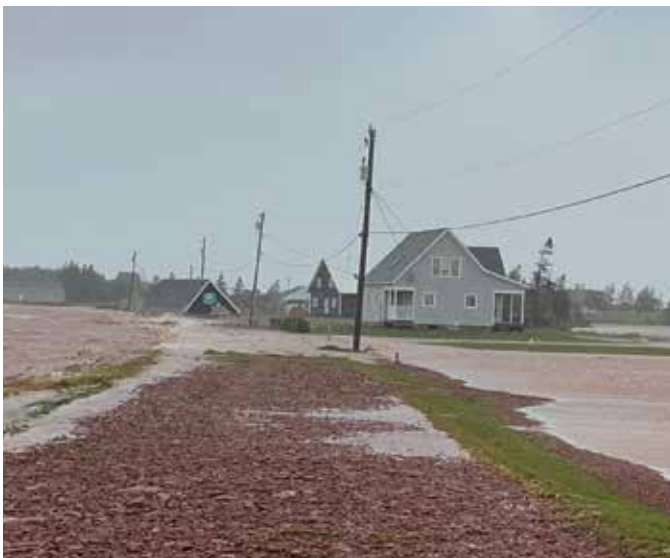
Figure 22. Storm surge flooding during Post-Tropical Storm Fiona, McEwan's Island, the Hebrides (shared with permission)
