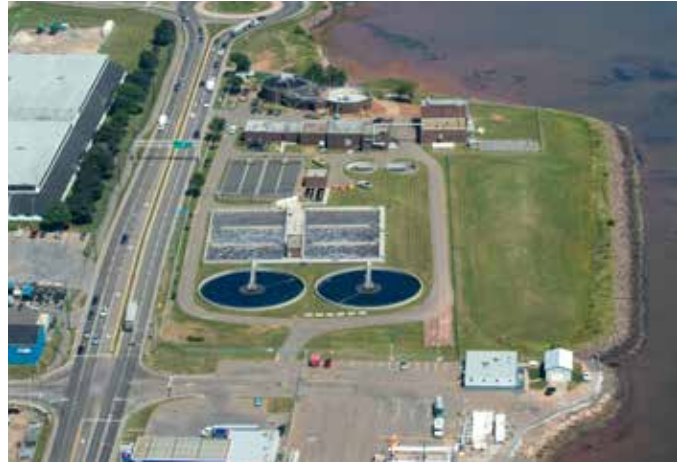
Figure 55. City of Charlottetown, Wastewater Treatment Plant, (D. Jardine, 2023)
