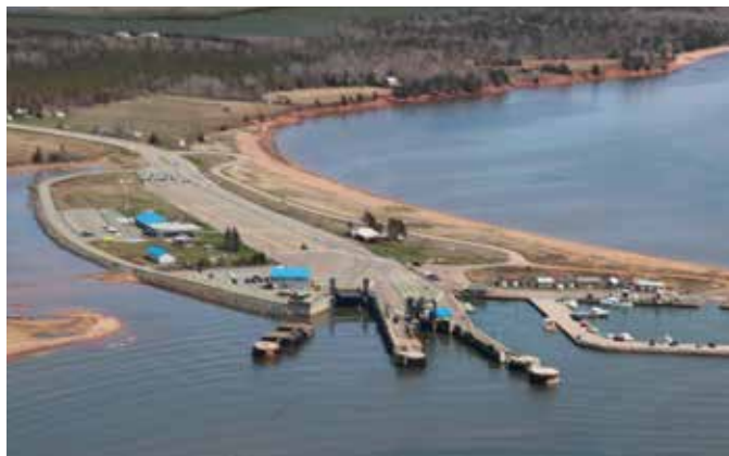
Figure 53. Wood Islands Ferry Terminal. (H Parnham, 2017)
