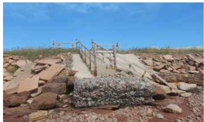
Figure 67. Beach access reinforced with poured concrete, concrete slabs and gabion baskets (H. Parnham, 2018)
