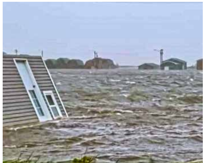
Figure 23. Building flooded by storm surge during Post-Tropical Storm Fiona. Malpeque Harbour PE (C. Wall, 2022)
