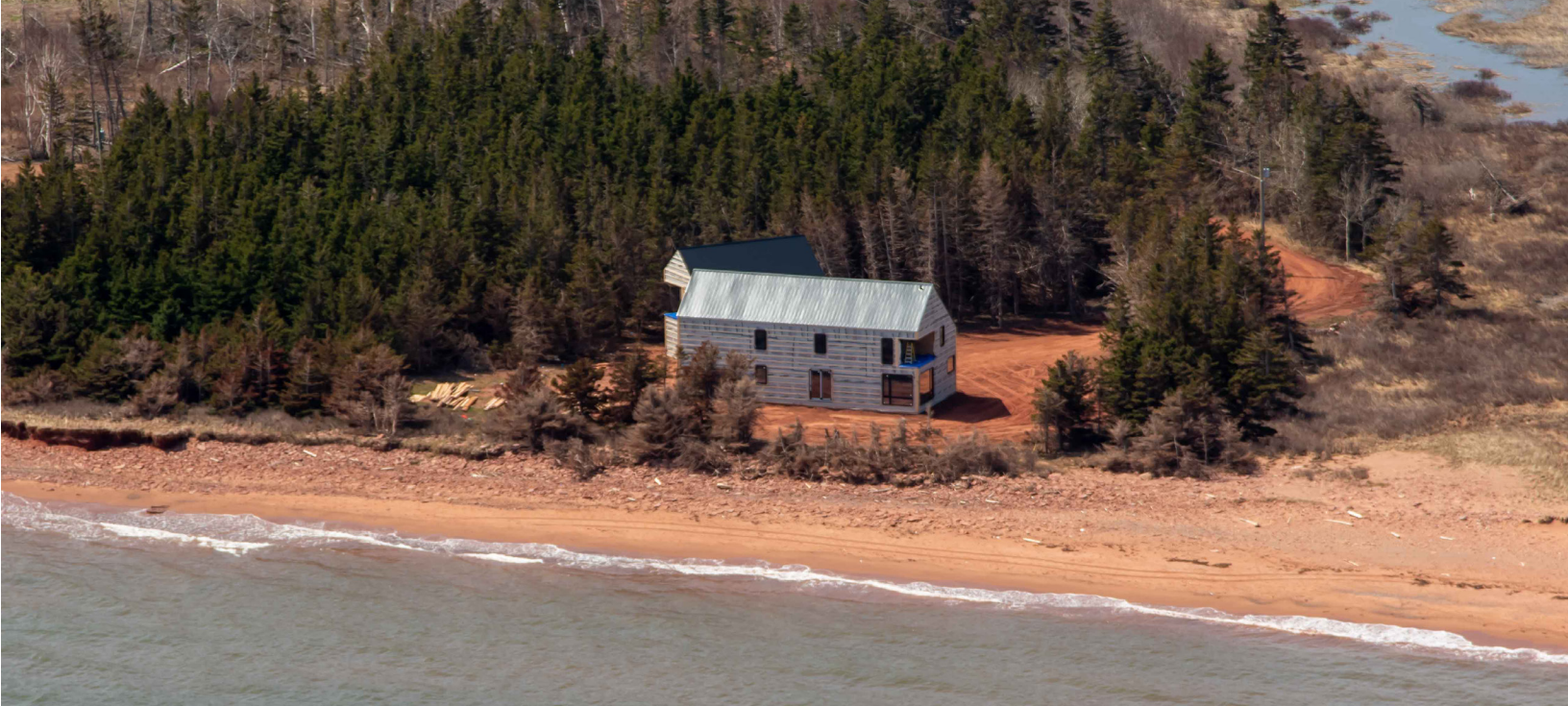
Figure 1. New residential construction on a low lying coastline surrounded by saltmarsh. Tignish Shore, PE. (D. Jardine, 2023)
