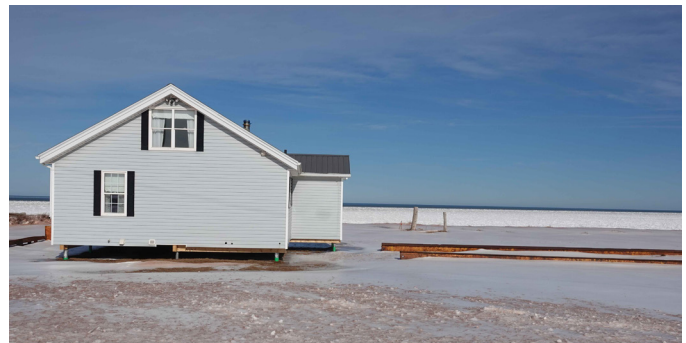
Figure 20. A house recently relocated and elevated. North Lake, PEI. (D. Jardine, 2023)
