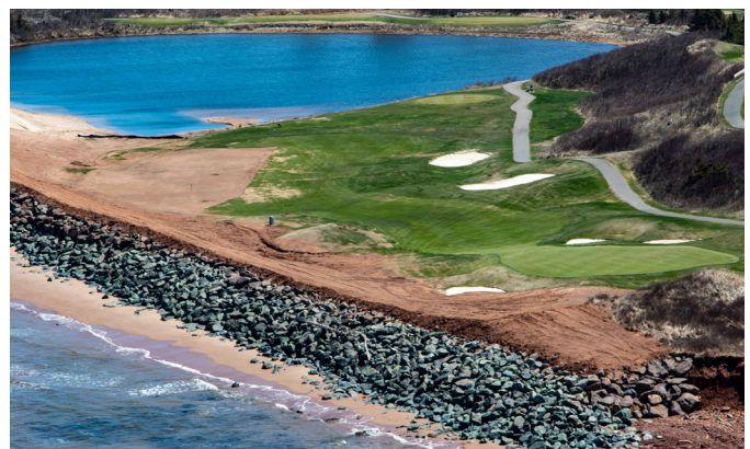
Figure 8. Coastal armoring installation at the provincially owned Links at Crowbush Cove golf course (D. Jardine, 2023)
