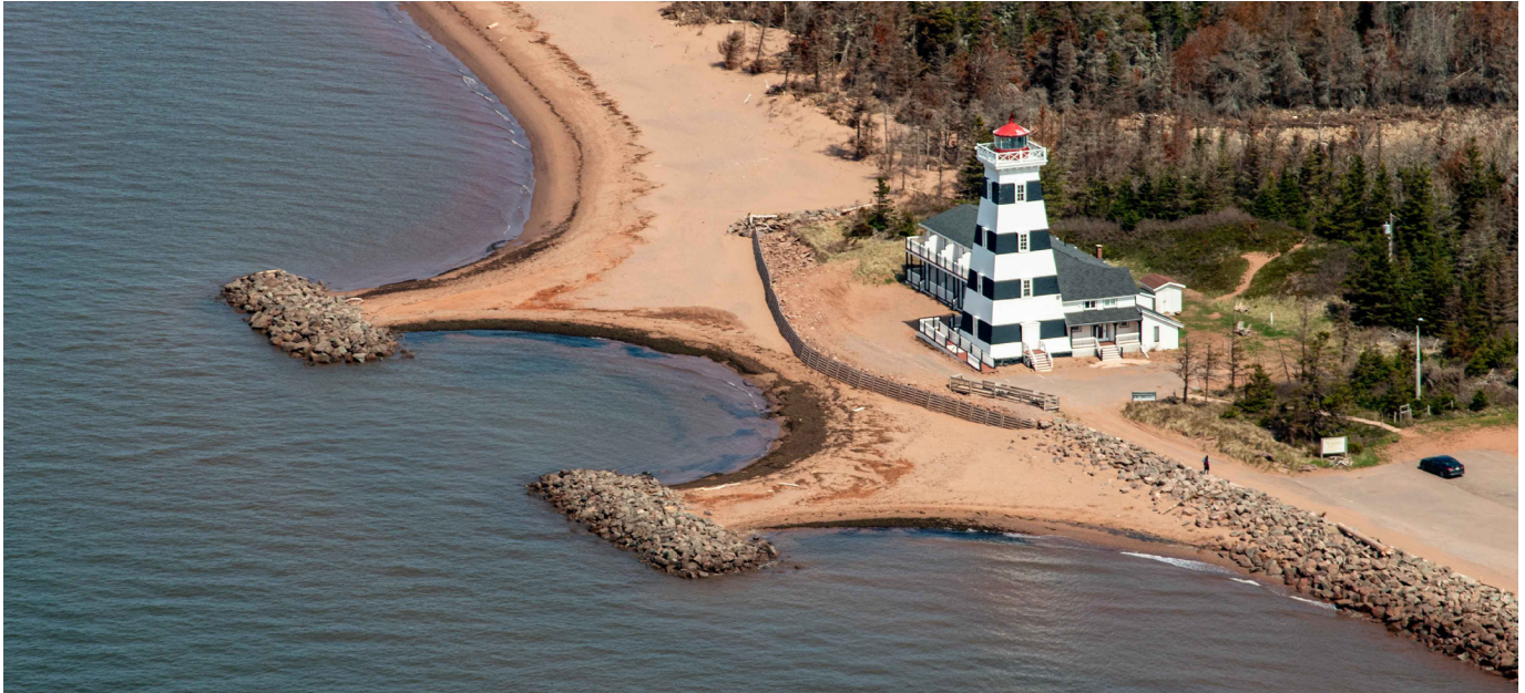
Figure 7. Artificial reefs for wave attenuation and sediment capture. West Point, Cedar Dunes Prov. Park, PE. (D. Jardine, 2023)
