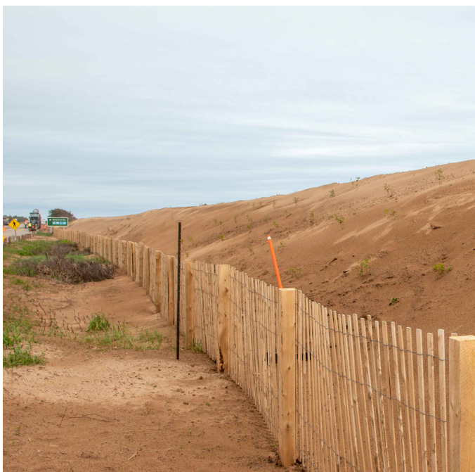
Figure 4. Buried revetment, sand renourishment and dune restoration. Dalvay, PEI National Park (D. Jardine, 2023)
