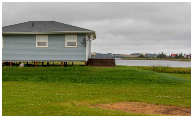
Figure 16. Following damage from Post Tropical Storm Fiona, this lot was raised 1.4 m and the cottage elevation raised to 3.7 m above mean sea level. As a cottage, this property was not eligible for financial assistance. MacEwen Island, PE (D. Jardine, 2023)
