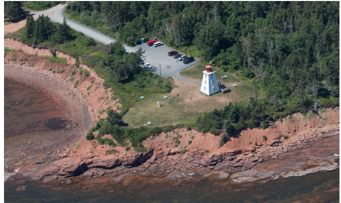
Figure 13. Cape Bear lighthouse in its new location. The structure was relocated from its original position in 2015 due to coastal erosion. Cape Bear, PE (D. Jardine, 2023)
